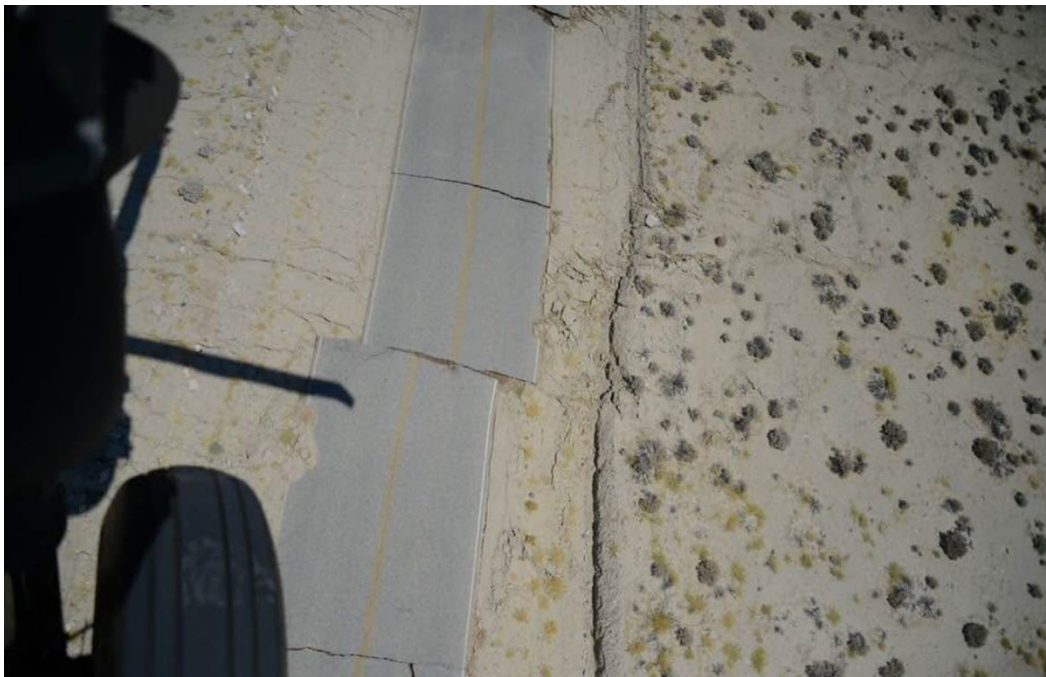
Figure 4 – Pretty hefty offset from the M 7.1 on the east-west road across the south side of China Lake playa (most famous 'anonymous' USGS photo that I ever took). Note the asphalt fractured ~perpendicular, not quite in line with the rupture zone; it acts like a rigid surficial plate breaks differently than the soil here. Note, too, the wheel and shadow are distinctive.
