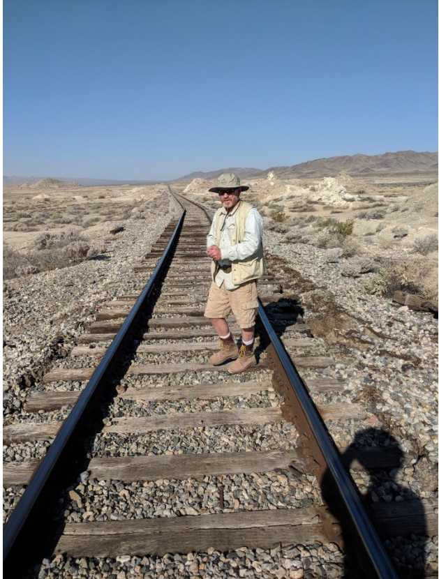
Train tracks deflected by the M7.1 rupture.
